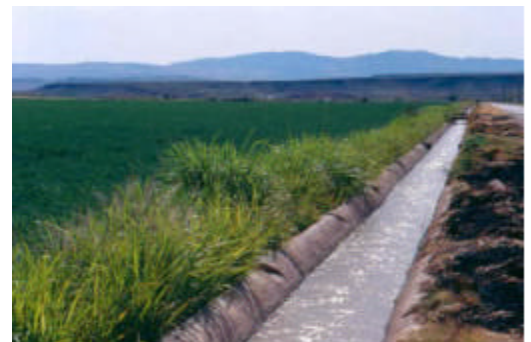
Concrete Lined Canal
